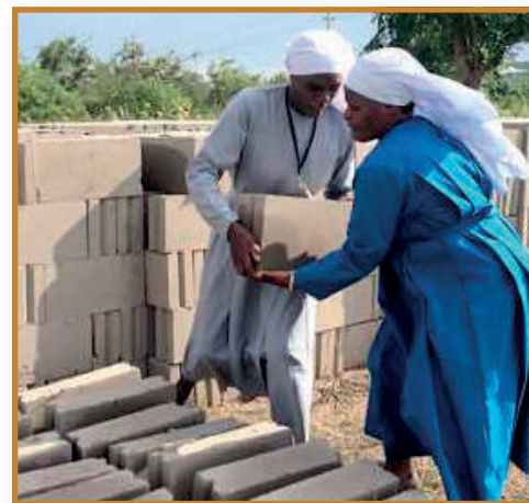
Stacking concrete bricks to build the school
