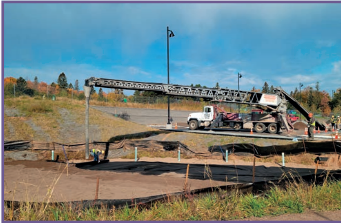
Retention basin being lined with layers of various soils
