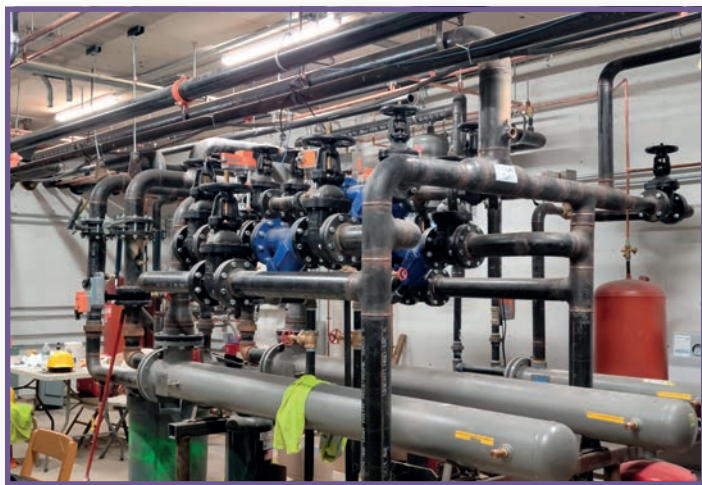
New mechanical equipment for distributing steam heat
