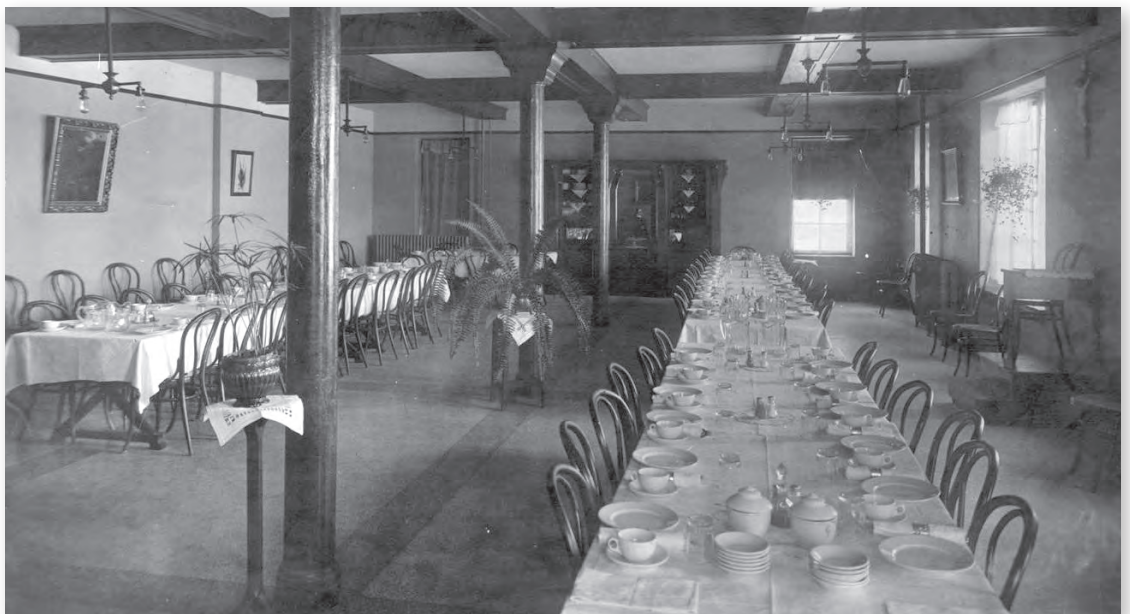
Student dining room showing the pillars and enclosed beams that were added to strengthen the building. Steel rods were strung below the ceiling in all rooms, except those of the fourth floor. The rods, covered by weathered oak, were artistically molded at the edges, giving them a look characteristic of the late Tudor style.
